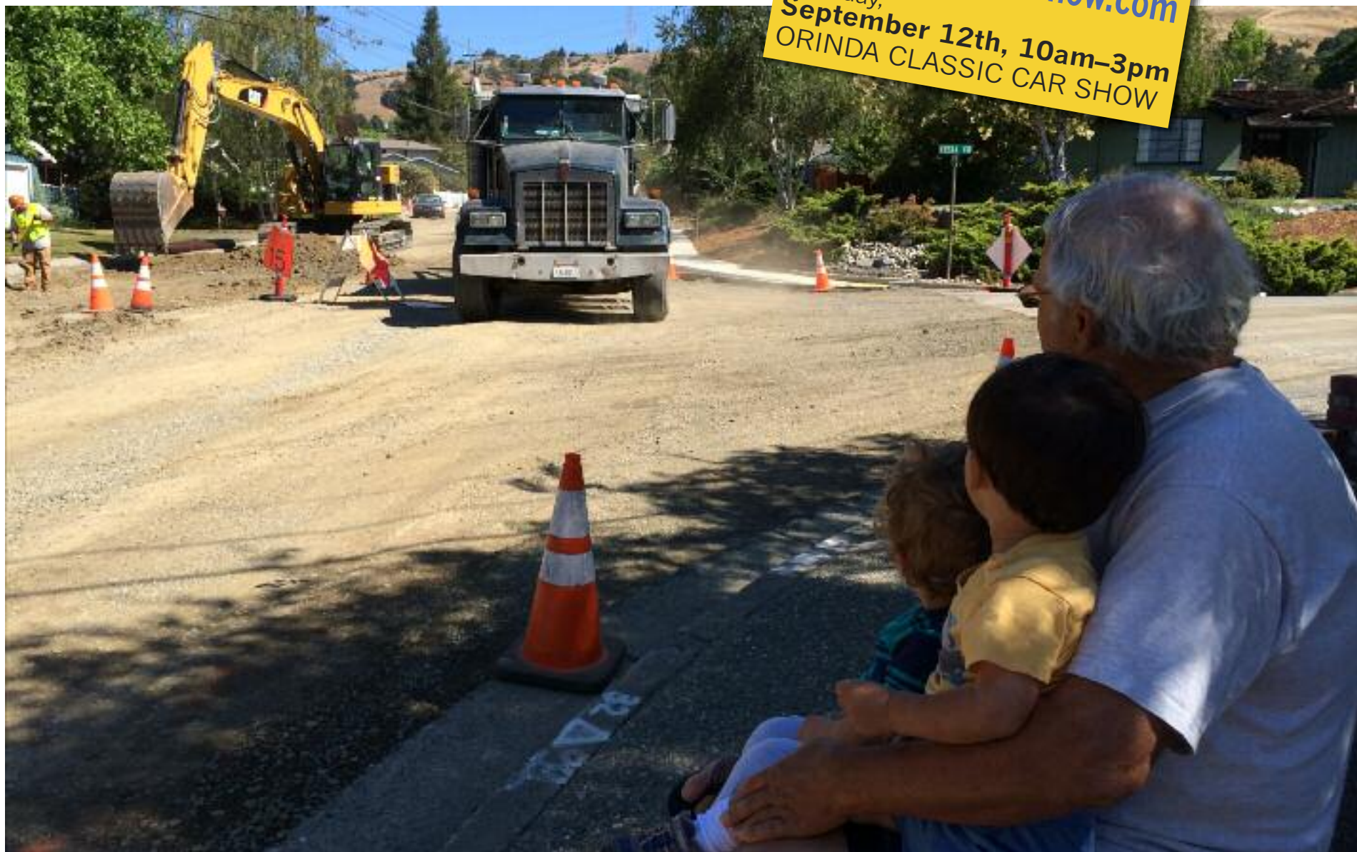
Vic Ryerson sits with his two enraptured grandsons as they watch construction vehicles at work on Ivy Drive in Orinda.
